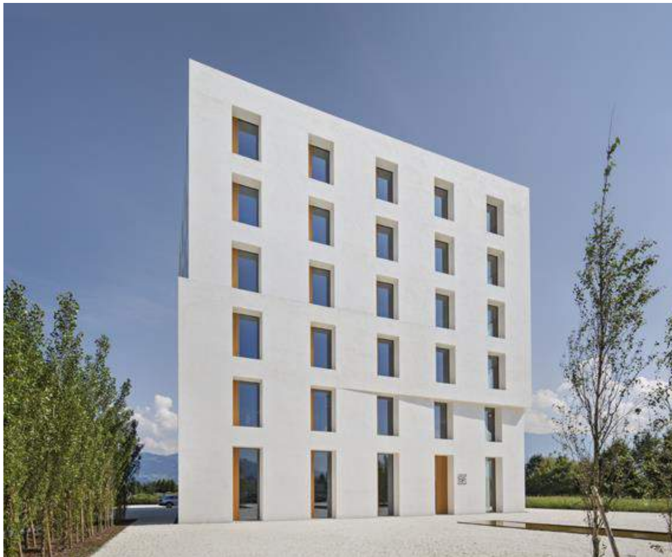
Arch. Baumschlager Eberle – Office building Lustenau (A)
